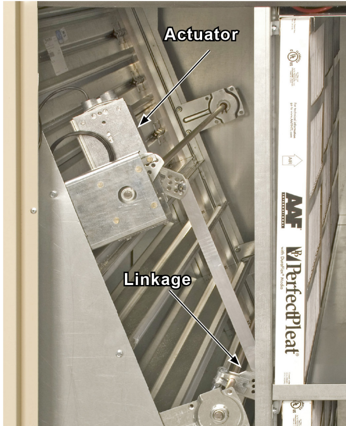
Figure 26: Damper Assembly
